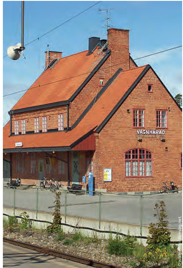
Vagnhärad station building
