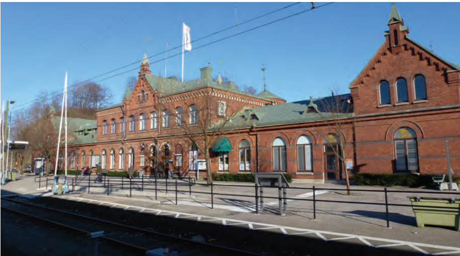
Borås station building - view from the platforms
